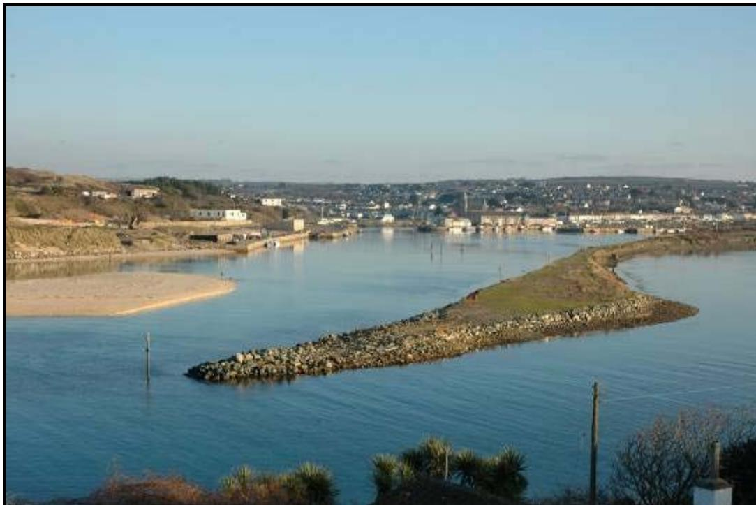
The Middle Weir also provides protection to Lelant from incoming waves during severe NW storms. During these storms significant amounts of sand are known to be moved and this can be readily observed within the Lelant SSSI where sand has built up.
